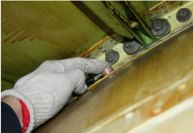
Fig. 5. The inspection with the ring type EC probe application.
